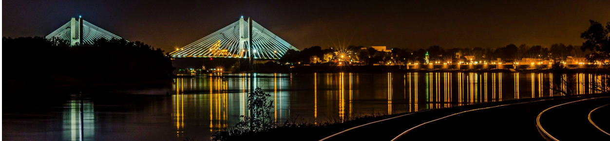
Figure 3.2: Night view of the Bill Emerson Memorial Bridge [6].
